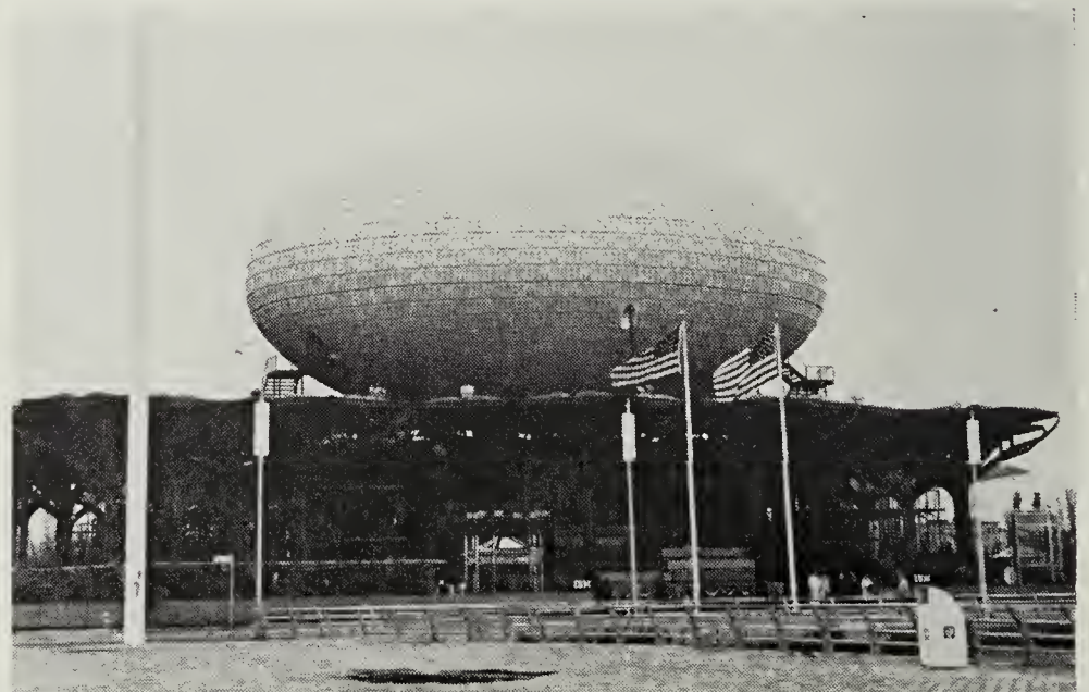
Sphere atop IBM building contains motion picture auditorium reached by inclined lift. Seven Simplex XL projectors are used in unique auditorium.
